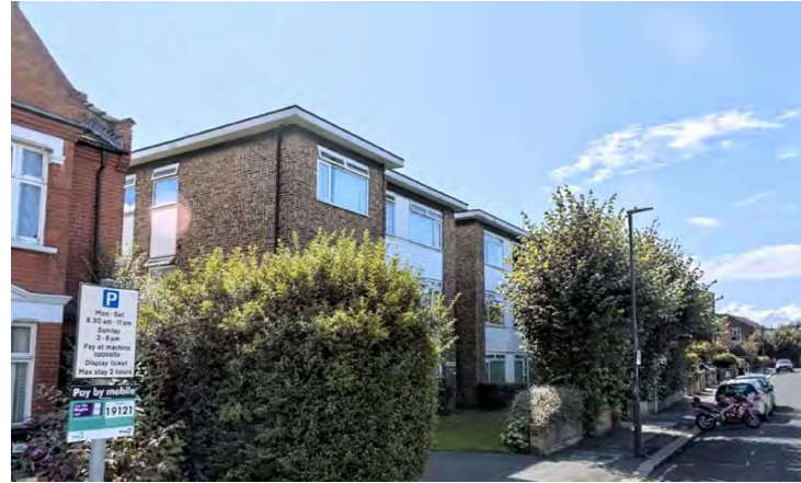
View of Site from Princes Road
